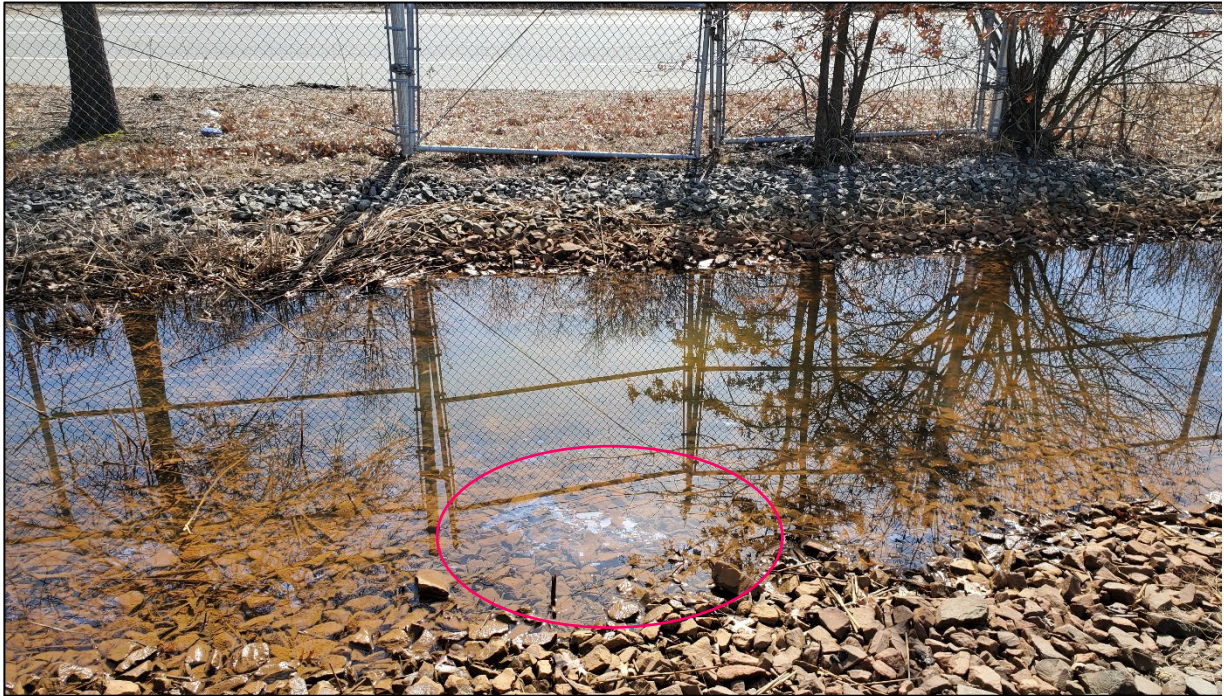
Photo 8. Possible depression in Eastern Drainage Swale at the northeast gate, limiting surface water discharge. No inlet grate or off-site discharge pipe present. Sheen in center foreground appears to be organic material, not petroleum.
