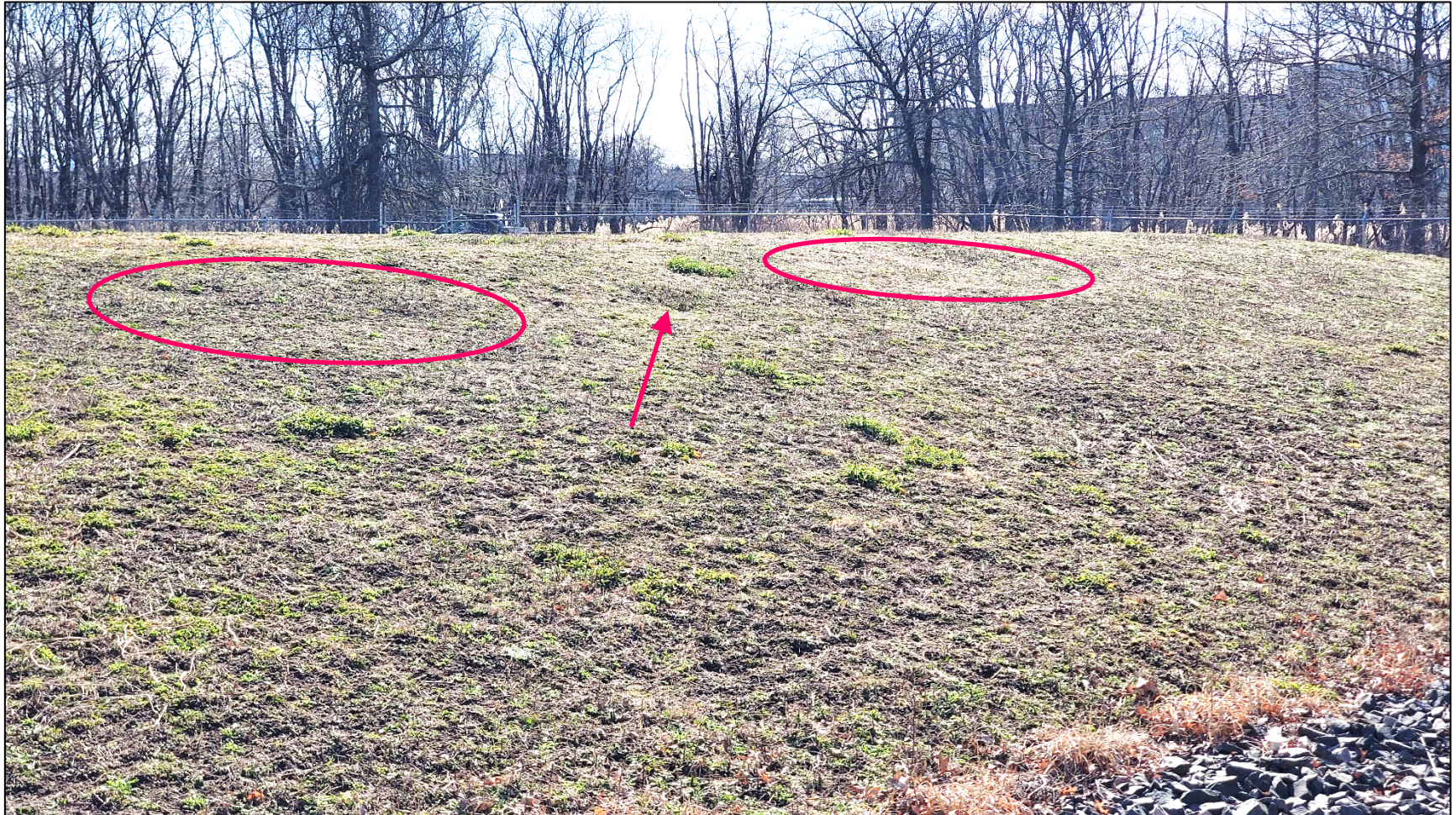
Photo 12. Southwestern portion of the soil cover showing minor depressions less than 0.9 feet deep. View is looking east.
