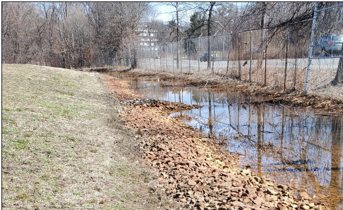
Photo 9. Leaf litter-clogged Check Dams within the Eastern Drainage Swale; some check dams appear to have had stone material removed from their centers to expedite surface water discharge.
