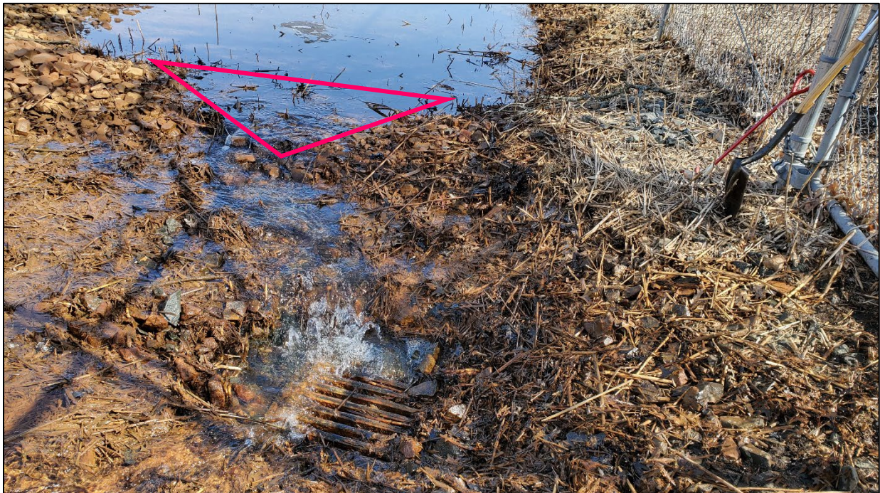
Photo 11. Eastern Drainage Swale Inlet Grate at the end of the site inspection. Triangle shows material removed from the upstream check dam, looking northeast.
